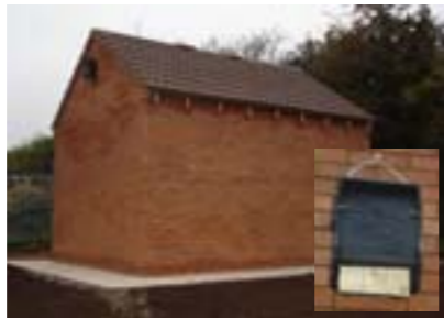
Severn trent's new bat house with (inset) its own bat box!
